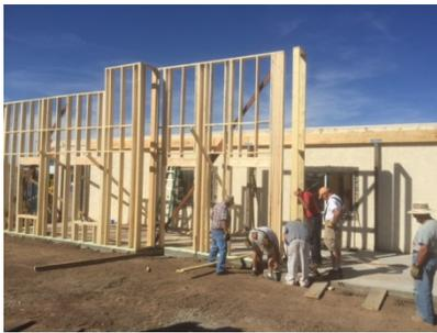
Ditches have been dug, sewer lines installed, footings dug, and what seemed like miles of rebar laid and tied. And none of all that work shows! Finally we were to the point of having concrete poured and putting up beams and raising walls. Weeks of work and the church can now see some results.
